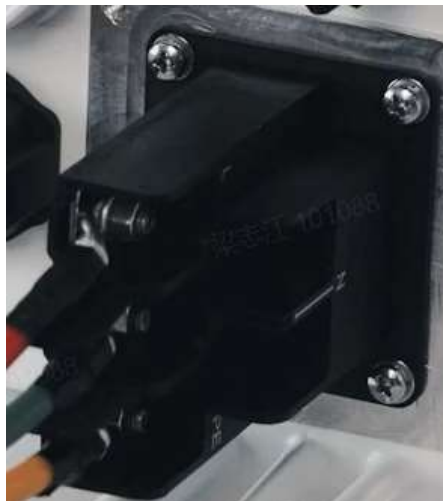
Image after installing the new AC Plug
